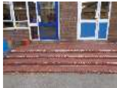
Below picture – additional handrail needed here.
