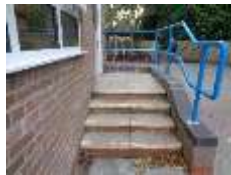
Below picture – additional handrail needed here.
